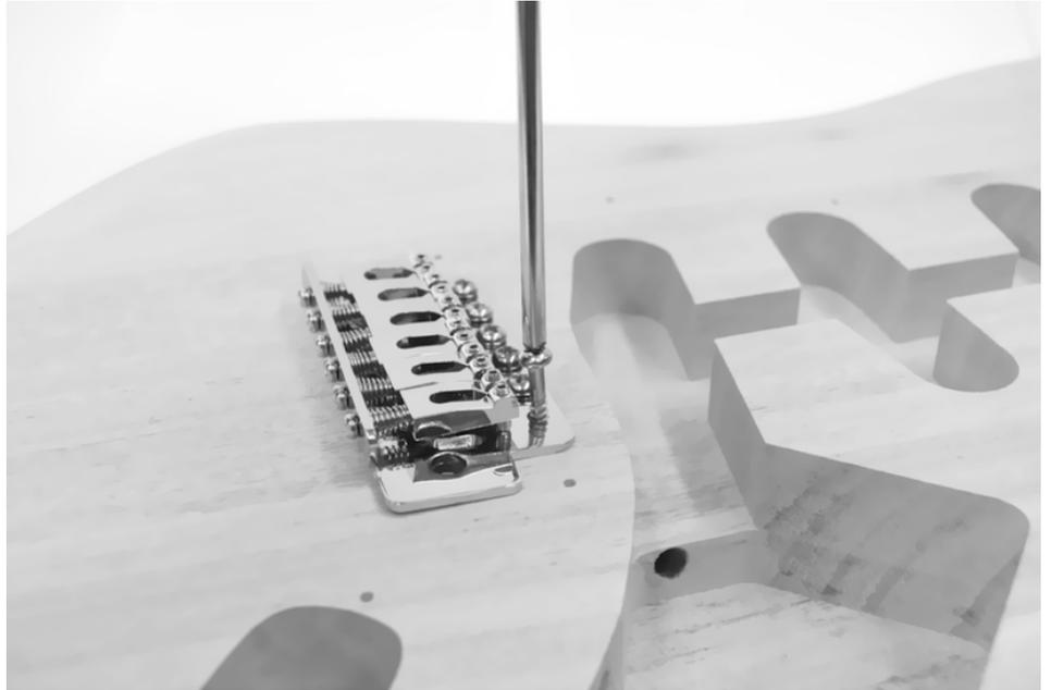
Next, turn the body around and screw the spring claw by hand into the pre-drilled screw holes in the cutout on the body's back.
