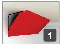
Fix one bracket to the ceiling and one to the wall. If using a corner trap, each should be 315mm from the corner. Note that the corner may be hidden behind the coving! If so just offer the trap up and mark it.
