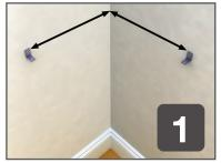
As per Section A, fix 2 L Brackets at the correct height to support the bottom edge of your trap. They should be located on adjacent walls, each 315mm from the corner.
